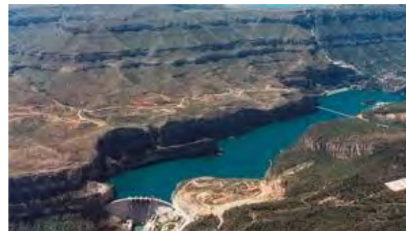
Foto: Muela Hydro (72 MW) plant
